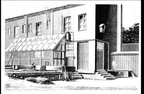
Large cast-iron solar hot boxes (numbered 1 through 10 in the diagram) built on the side of Charles Tellier's Paris workshop. The thick metal plates were needed because the working fluid was ammonia under pressure. Tellier hooked up the pump powered by the ammonia to lift water from his well. Two iron sheets riveted together to form a watertight seal. Ammonia was used as a working fluid under pressure, because of its lower boiling point.
