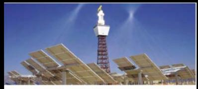
During daylight hours, 2000 mirrors at Solar Two track the sun and store its energy as heat in molten salt. This energy can then be used to generate electricity when needed, such as during periods of peak demand for power.
