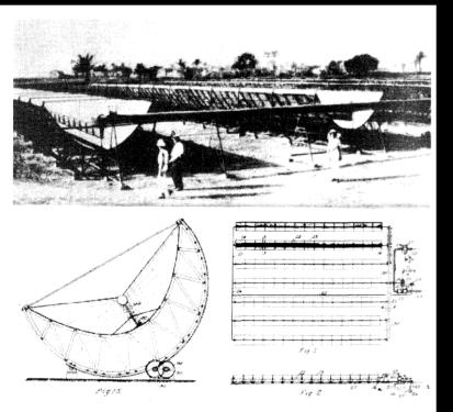
Frank Shuman's Maadi plant in Egypt, with cutaway diagram of the parabolic trough collectors.
