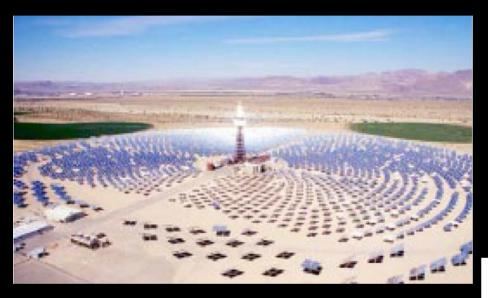
**Power Output:** Solar Two produced 1633 MWh over a 30-day period, exceeding its one-month performance measure of 1500 MWh of power production; the plant also produced a record turbine power output of 11.6 megawatts.
